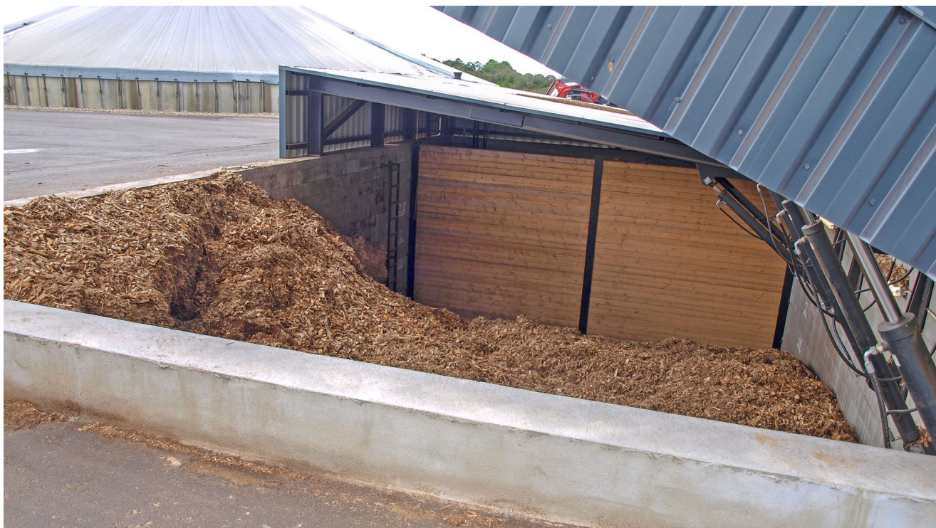
Figure 3-11: Biomass Delivery Bunker (Lin-Ka Energy)
