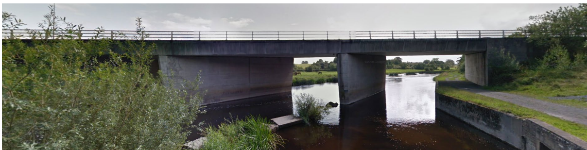
Figure 3-21: Cardinal Moran overbridge river view
