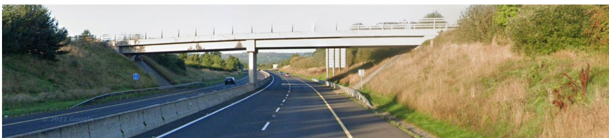
Figure 3-17: Location of L3038 Overbridge across M9 Motorway View
