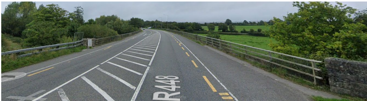
Figure 3-20: Cardinal Moran overbridge street view
