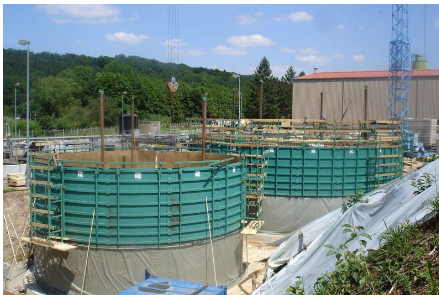
Figure 3-32: Climbing Concrete Formwork (RSB formwork technology, 2026)
