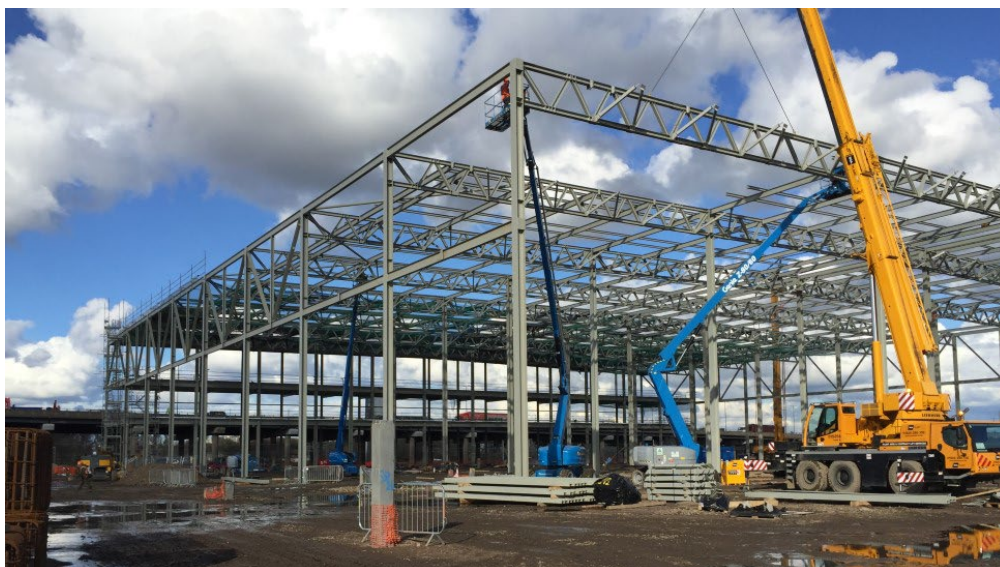
Figure 3-26: Steel erection: Crane and Mobile Elevated Work Platforms (Wall Steel, 2026)
