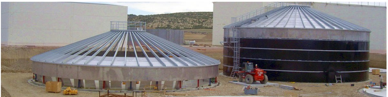
Figure 3-31: Digester Tank Construction (Biogas Consulting , 2026)
