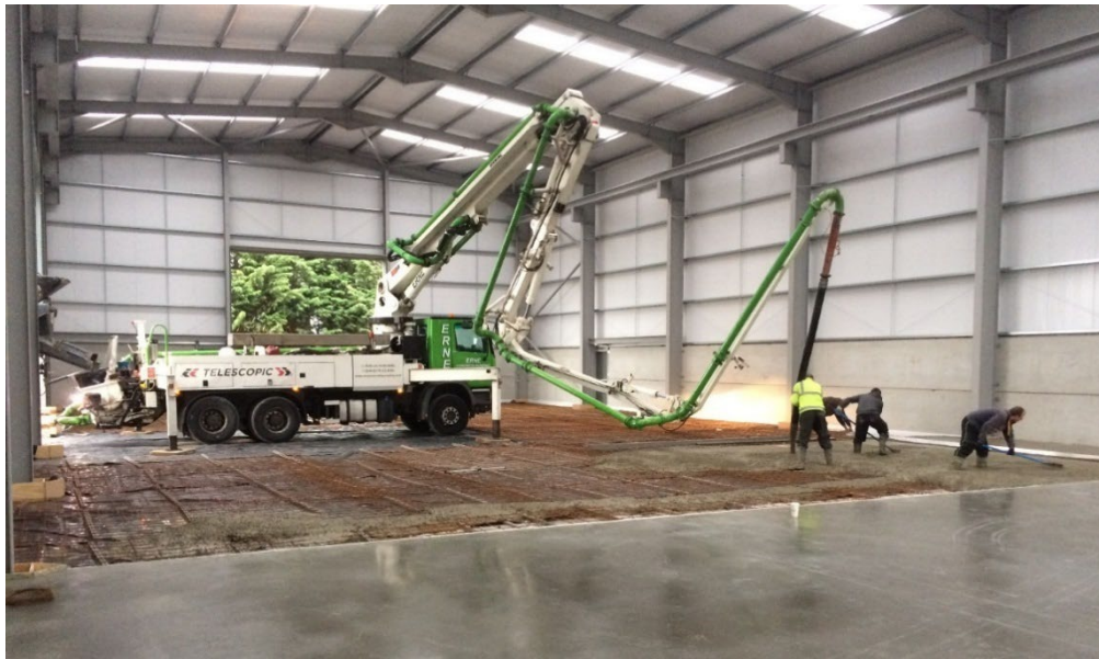
Figure 3-28: Placement of Reinforced Concrete Floors (Concrete Pumping Ltd., 2026)
