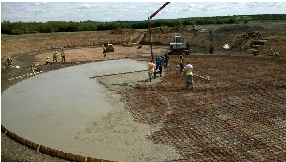
Figure 3-29: Construction of Digester Tank Foundations (BioWatt, 2026)
