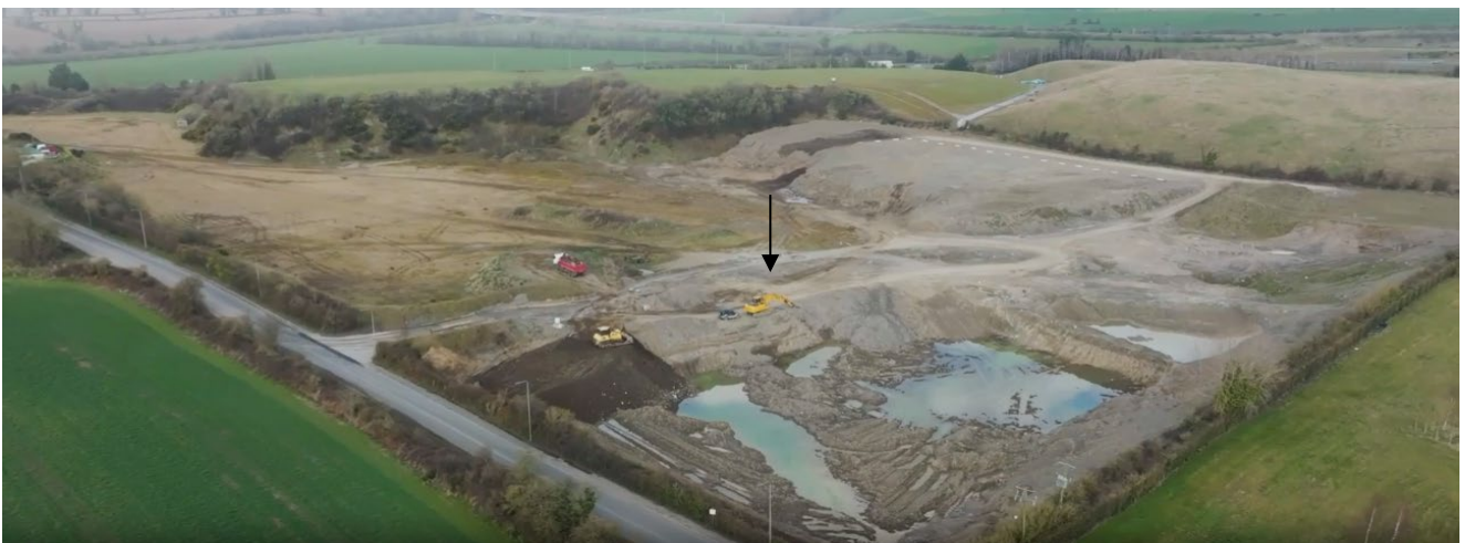
Figure 3-3: View from southeast (active quarrying in foreground)
