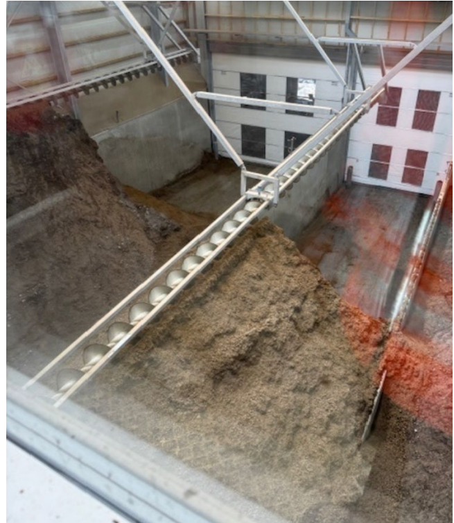
Figure 3-10: Solid Digestate Elevated Conveyor System
