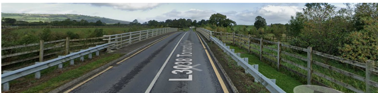
Figure 3-16: Location of L3038 Overbridge across M9 Streetview
