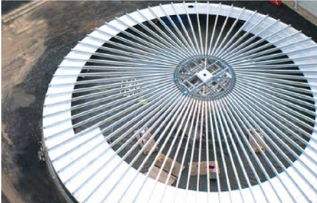
Figure 3-30: Stainless Steel Roof - Ground Level Construction (Balmoral Tanks, 2026)
