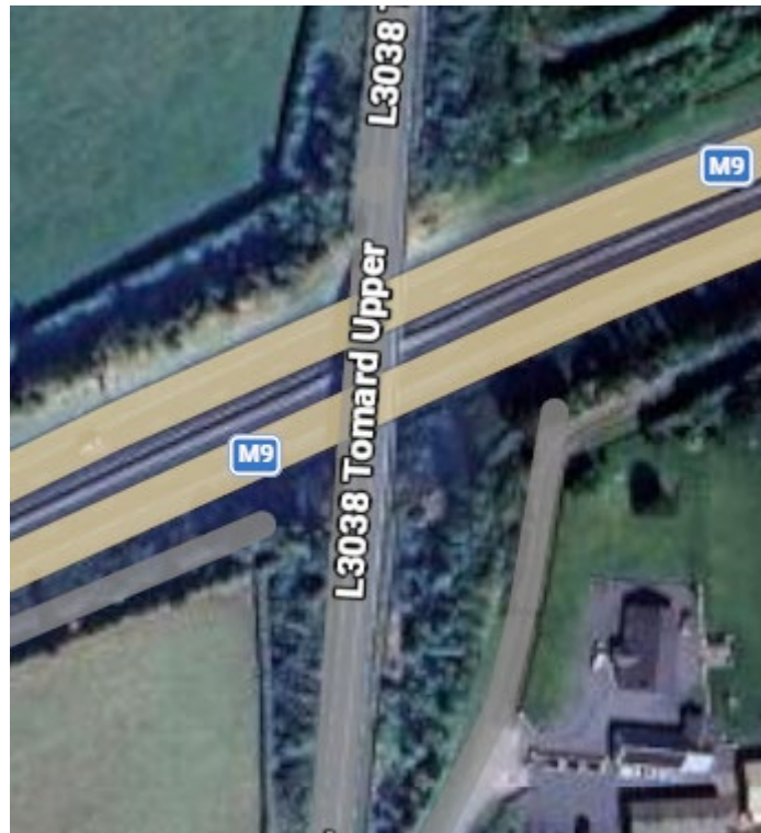
Figure 3-15: Location of L3038 Overbridge across M9 Aerial View
