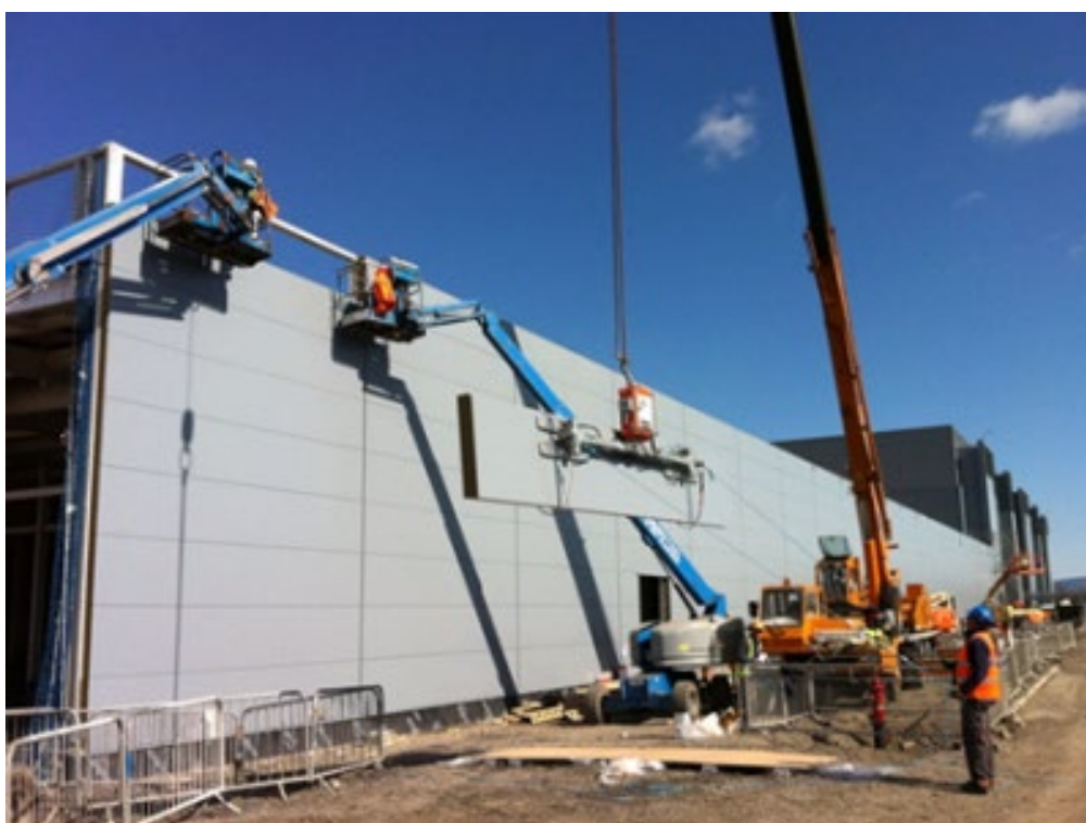
Figure 3-27: Cladding Installation Portal Frame (Steel Construction Info, 2026)
